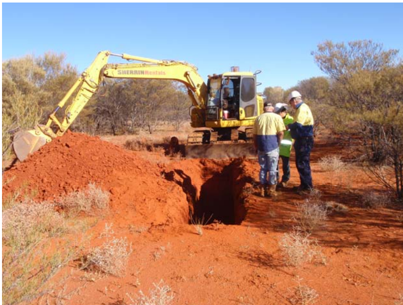
Geotechnical test pit excavation at the site of the Nolans process plant
