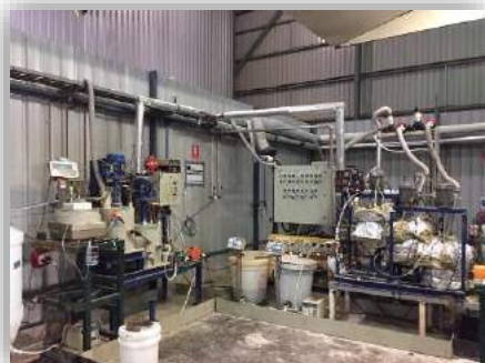
Phosphate Extraction Pilot Plant
