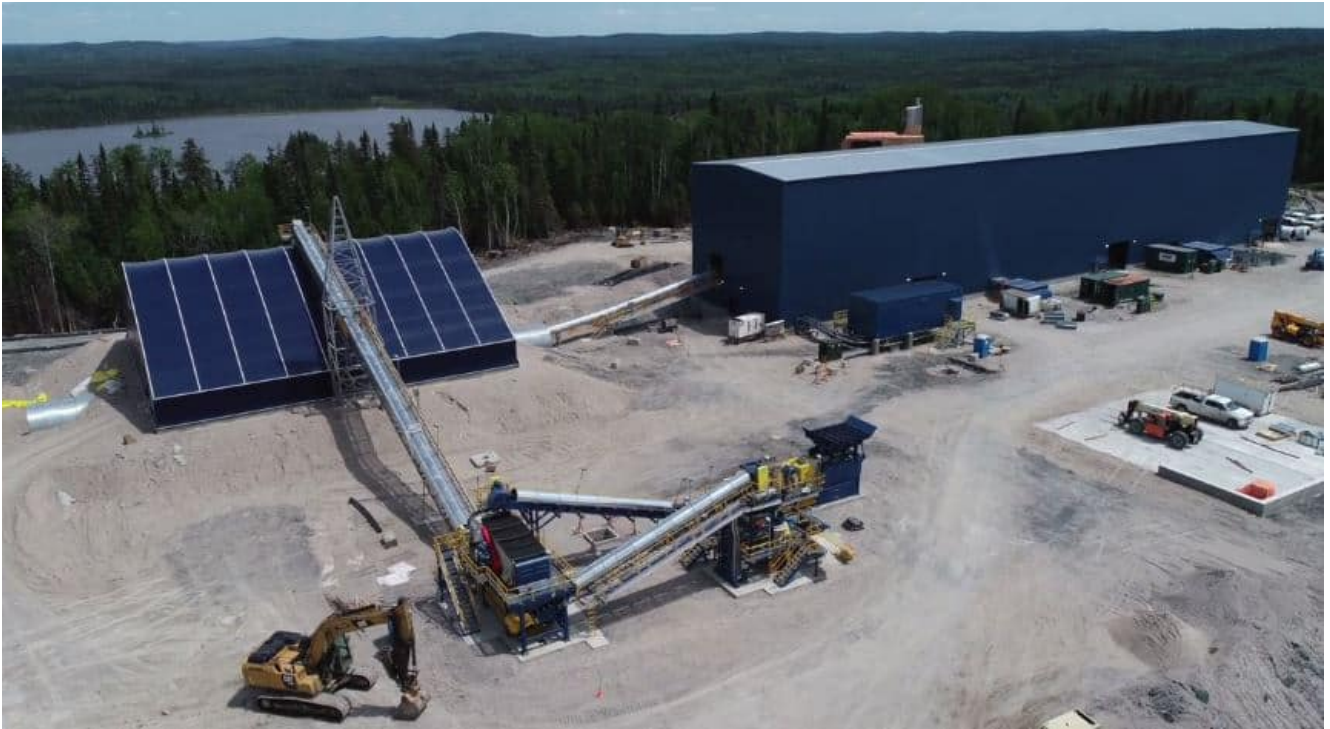
Sugar Zone crushing plant
