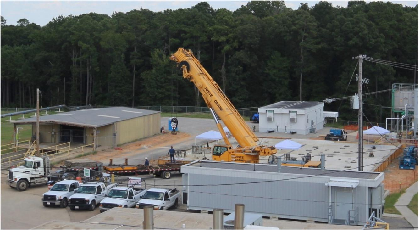
*Project Site Location Showing Completed Foundations and Mobile Crane Ready to Install Modules – Image taken Aug 21st, 2019*
