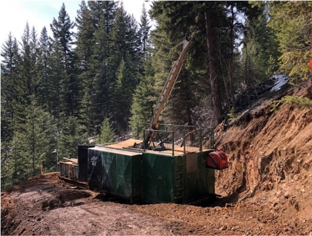
Figure 2: 2021 Drilling at Gate Zone, MPD and Core Logging Facility, Merritt BC
