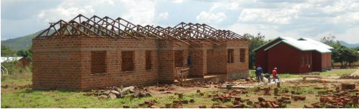
Figure 2: Construction of a second duplex house for Ngwala Primary School teachers. The first duplex completed earlier in the 2013 can be seen in the background.
